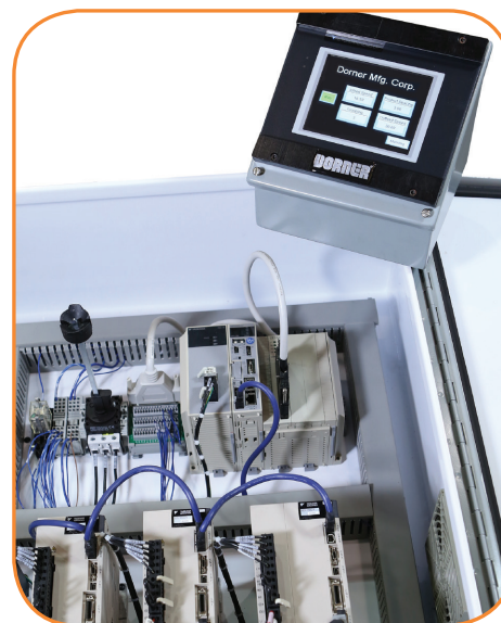
Control Box with HMI
