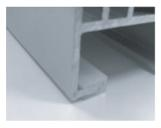
Make sure the slide rail is proper mounted and snaps onto the beam. Please identify that the longer flange of the slide rail must always face inner of the beam.
